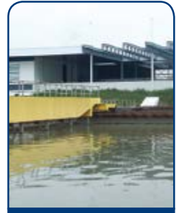
Wastewater Treatment Plant, Lyon, France, Large Diameter
